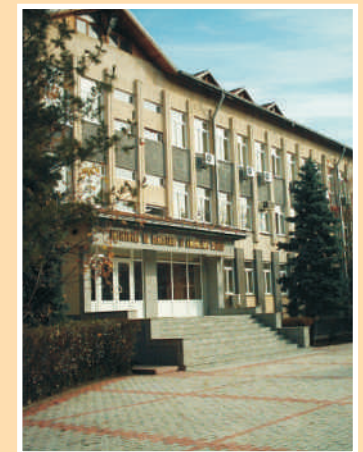
The present headquarters of ICAS (1976, transferred from 46 Pipera Av., Bucharest) 128 Eroilor Blv., Voluntarii
